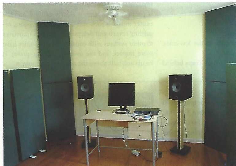
Fig. 3. Room treatments from GIK Acoustics are brought in to help tame the reflections.
